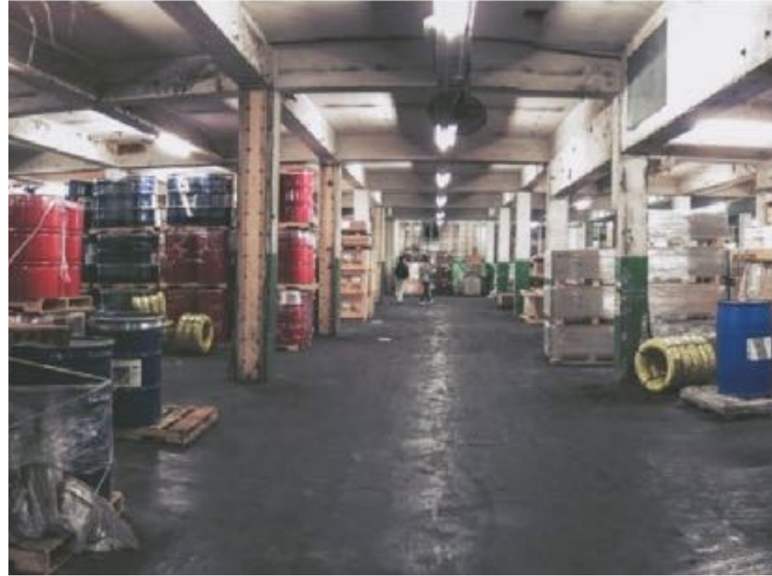
The Hall before reconstruction 未活化前的紗廠坊
