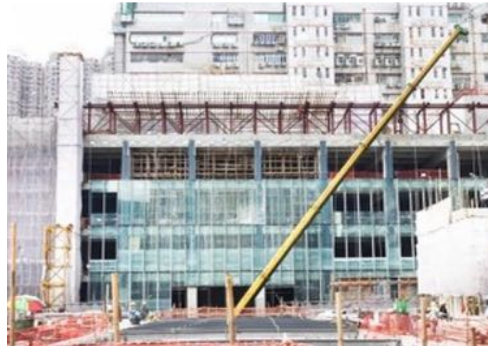
The glass wall during reconstruction 正在施工的玻璃幕墙
