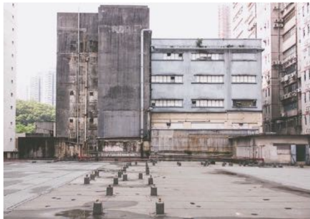
The Deck before revitalization 未活化前的紗廠耕地
