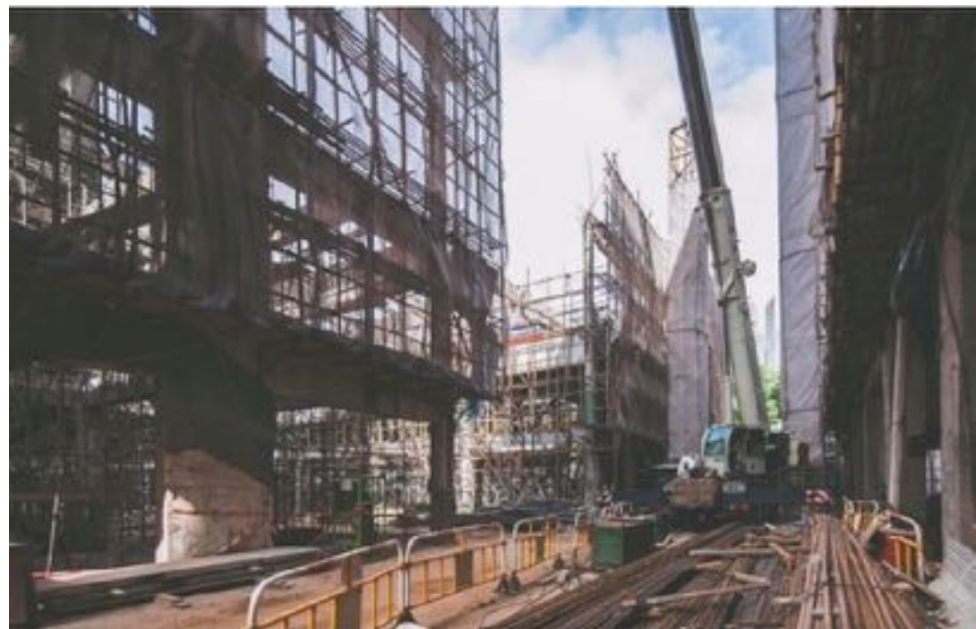
Before the construction of the Glass Link Bridge 施工前的玻璃橋
