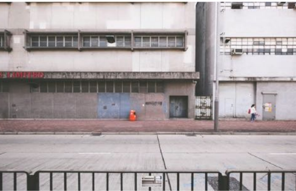
NF5 Gate before revitalization 五廠鐵閘
